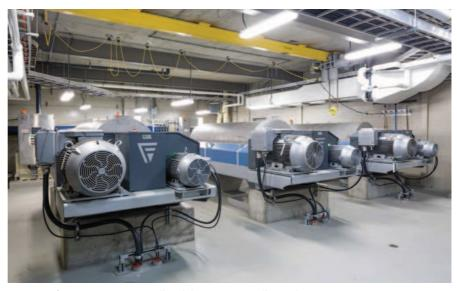
Two centrifuges operate continually, while one is in standby mode.
