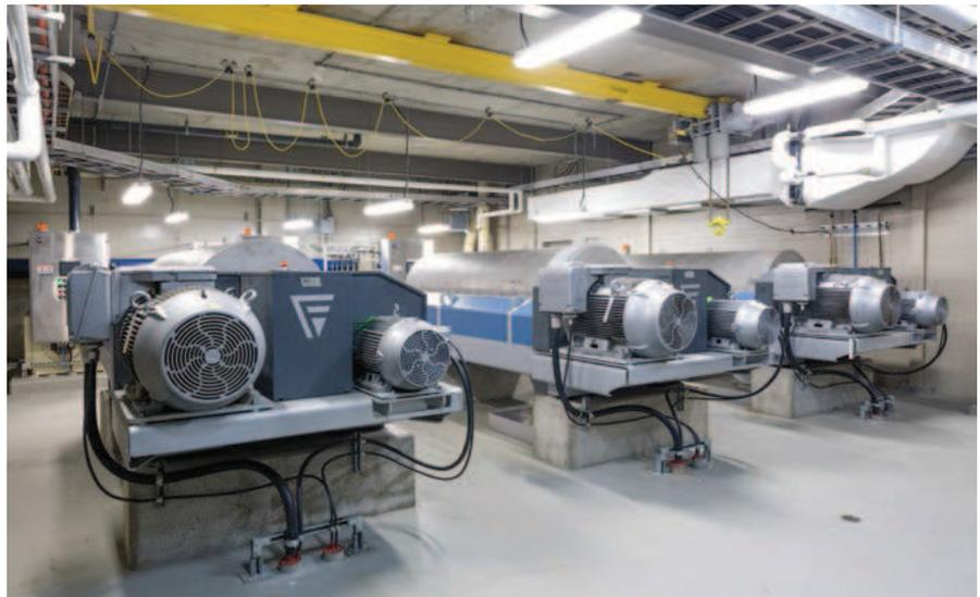
Two centrifuges operate continually, while one is in standby mode.
