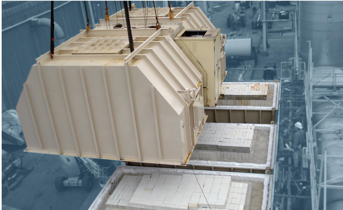
INSIDE STORY: As ethanol plants reach the 10-year mark, the ceramic media inside the regenerative thermal oxidizer can become plugged and need replacement.
