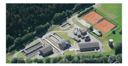
Because of the geographic situation (upstream of the dam) it is necessary to keep the phosphate discharge concentration below 0.2 mg/l, which is only possible using flocculation filtration. As a consequence, the sludge quantity increases by 10 %. Since the end of 2008, the entire sludge has been dewatered using a Flottweg decanter of the new **C series.**
